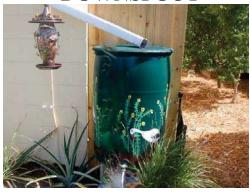
Cut or remove a portion of your downspout to divert water from your roof into the rain barrel
