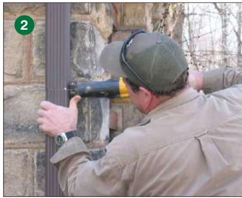
Cut off an existing downspout above the barrel.
