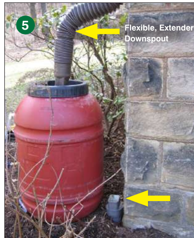
This set up allows the downspout to be re-attached, and the barrel stored in winter.
