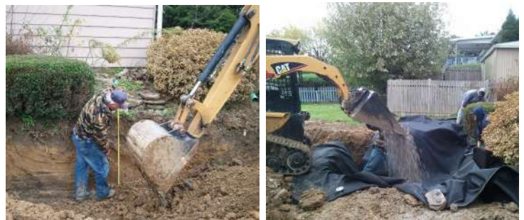
Digging and backfilling a dry well for a roof downspout.
