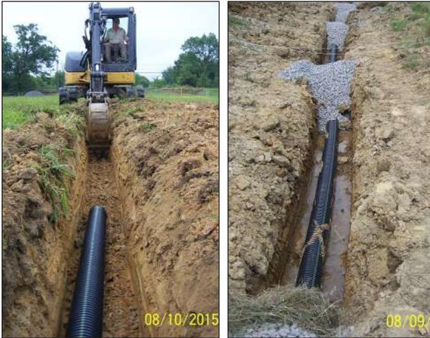
Trenching and backfilling an underdrain
